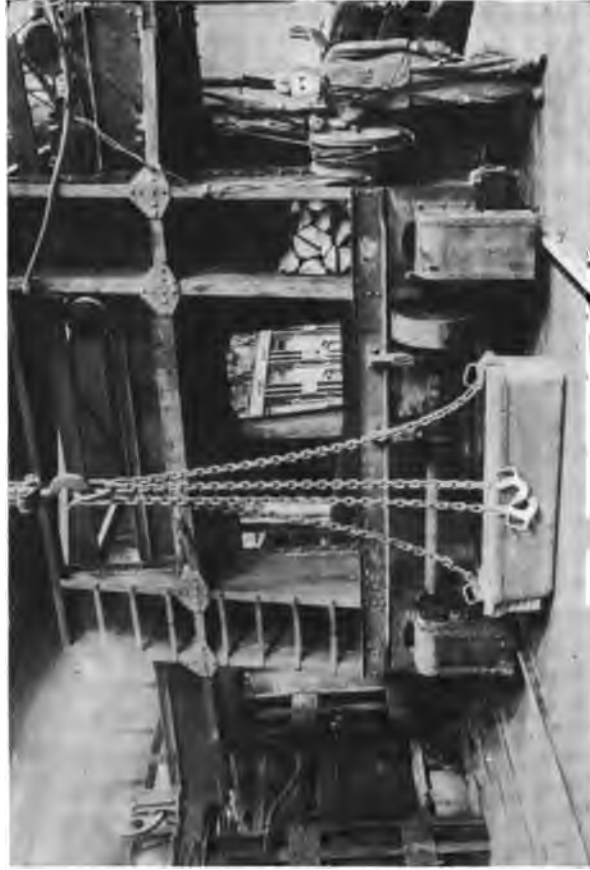
Fig. 1. Footwalk on Outside of Open-Hearth Building, giving access to Crane Runway within. (American Steel and Wire Company.)*
